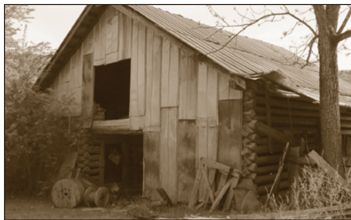
Underneath its rough tin skin, the Beck Barn is an impressive four-pen, crossed-hall log structure with a massive overhead loft. The barn was donated to Foxfire this spring, and will be taken apart, moved to the Museum, and reconstructed, hopefully to become display space for older and recently-acquired farm equipment.
